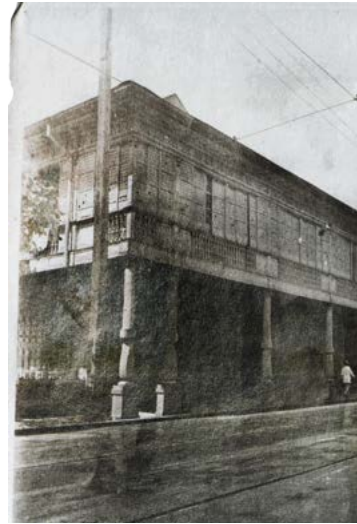
"Casa Grande," 964 R. Hidalgo Street (former Calle San Sebastian) © TLC
